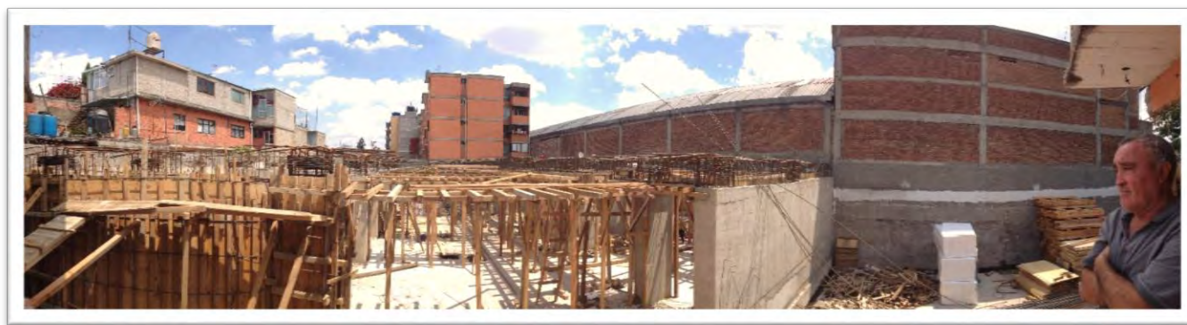
Photo 6: The construction site under the scrutinizing look of the engineer.
